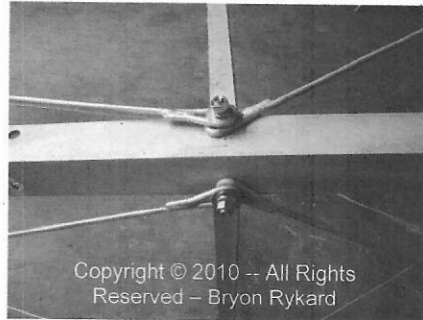
Figure 6b: Close up of the assembled girt and short and long flat strap "X" bracing (top view) NOTE: These are round rod braces in lieu of the flat strap braces on most WindEngine Towers
