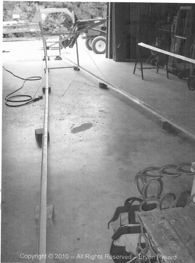
Figure 8: All the upper corner posts, girts, and "X" bracing assembled with 2 lower corner posts.
